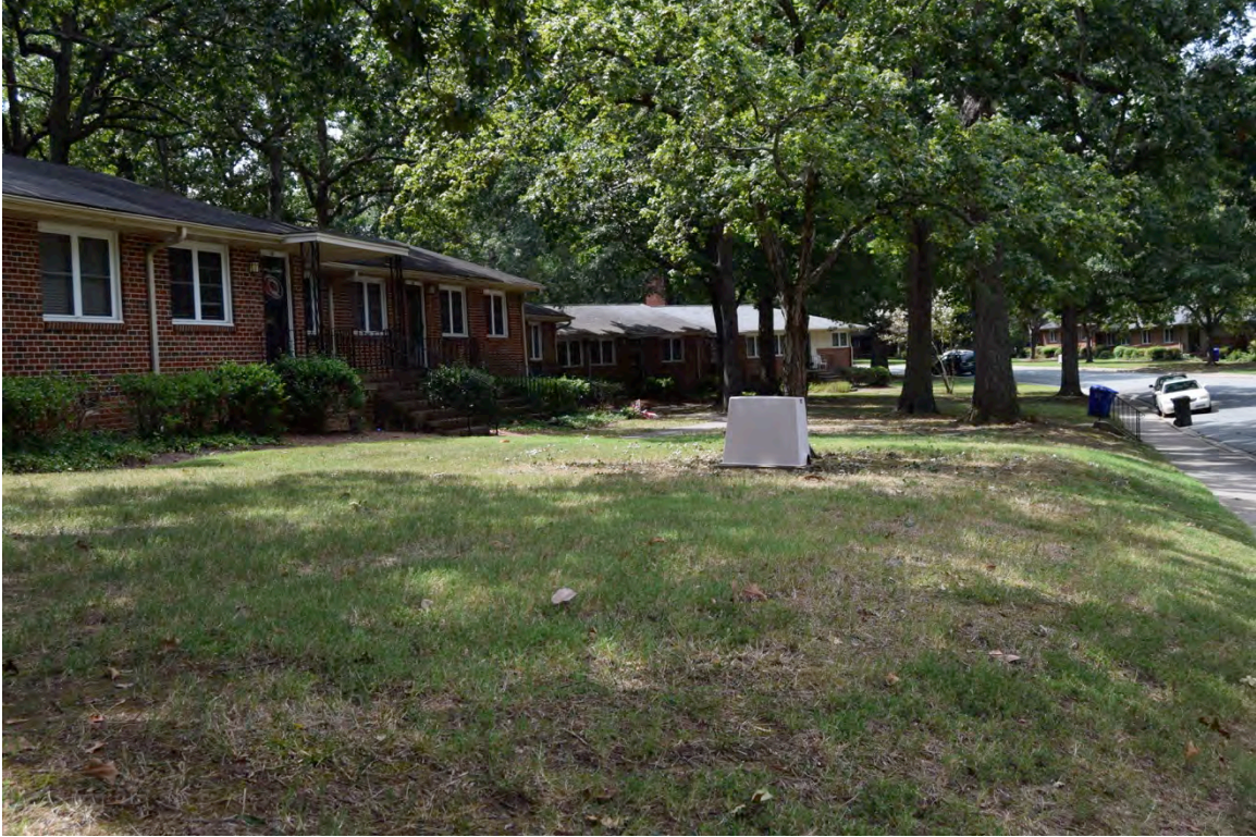
Figure 13. Glen Lennox Superblock apartment buildings extending west from Maxwell Road, view southwest.
