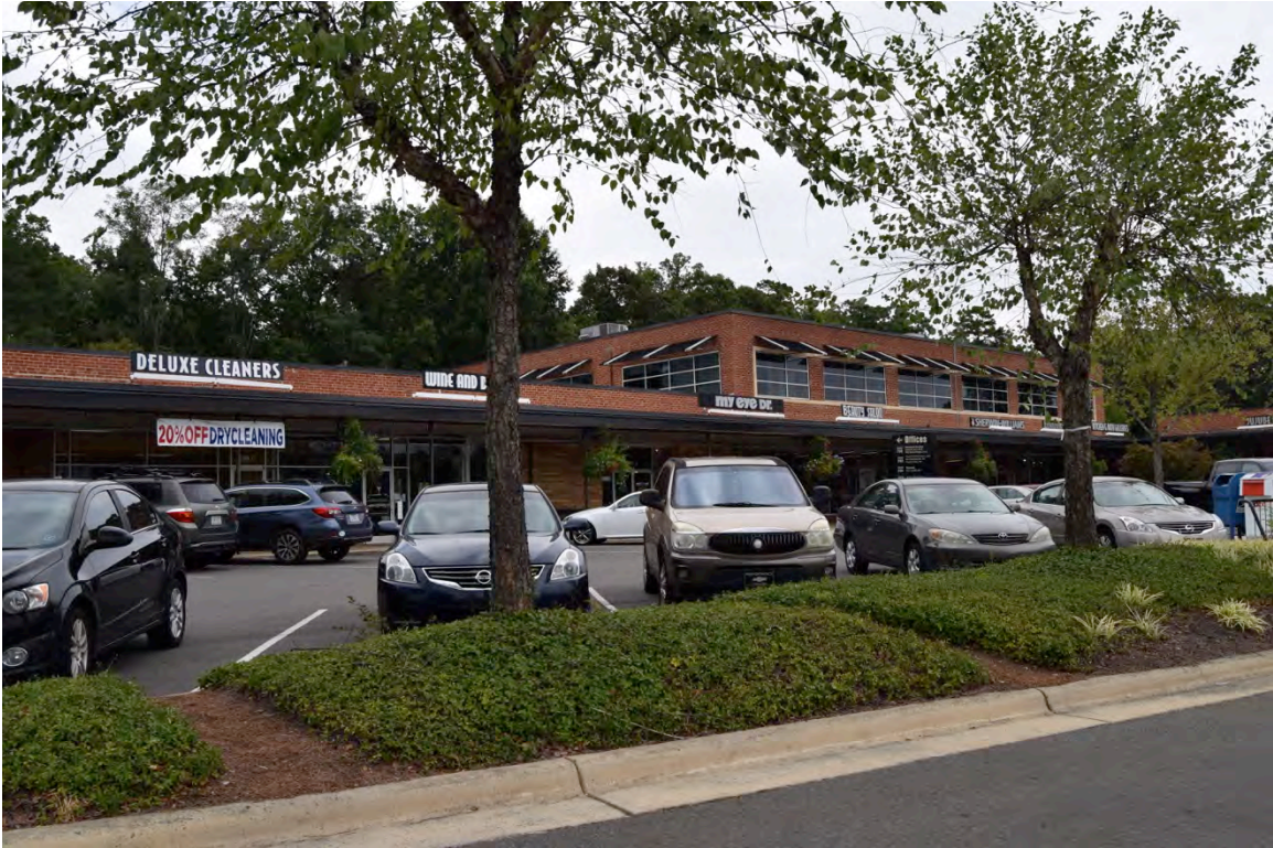
Figure 10. Glen Lennox Shopping Center, view to northeast.
