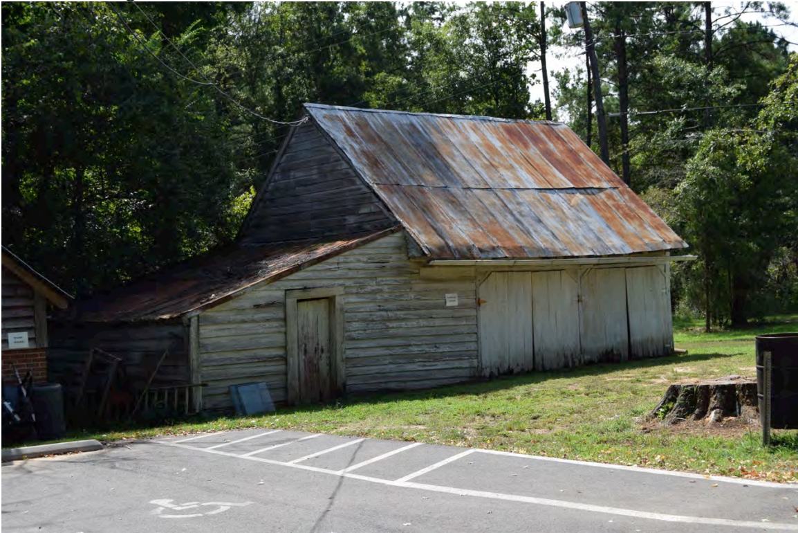
Figure 46. Carriage House, Leigh Farm, southeast
