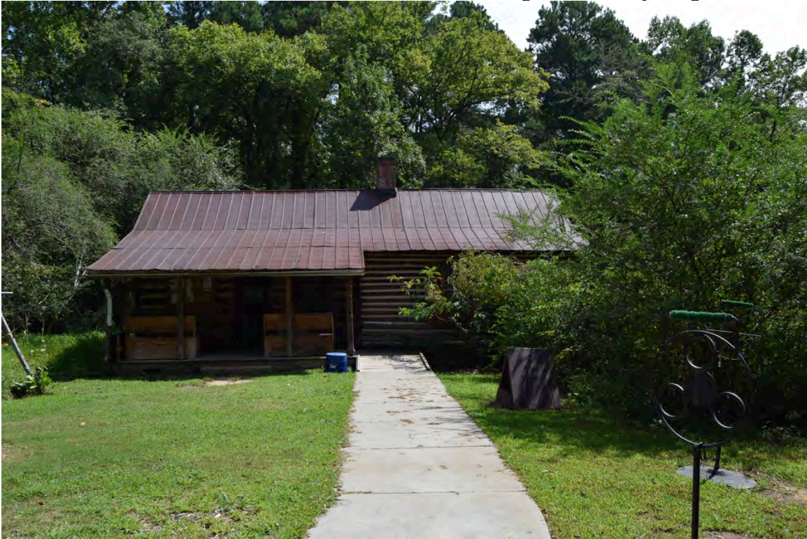
Figure 45. Enslaved People's Dwelling #2, view east
