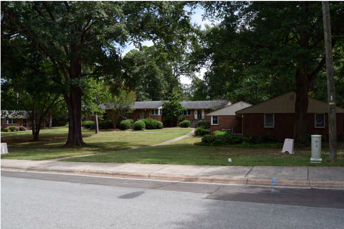
Figure 12. Glen Lennox Apartment Superblocks on east side of N. Hamilton Road, view to northeast.
