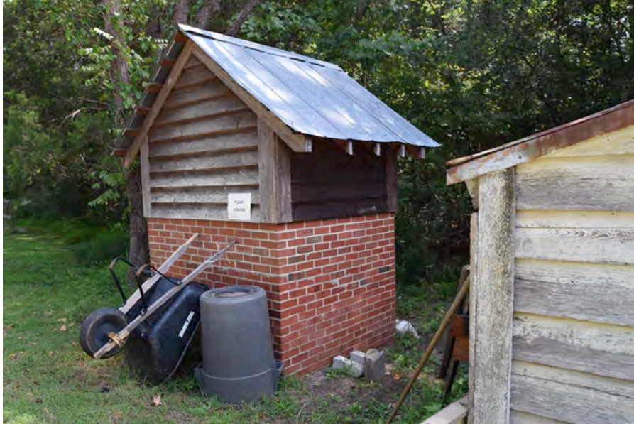
Figure 49. Pump House, Leigh Farm, view west.
